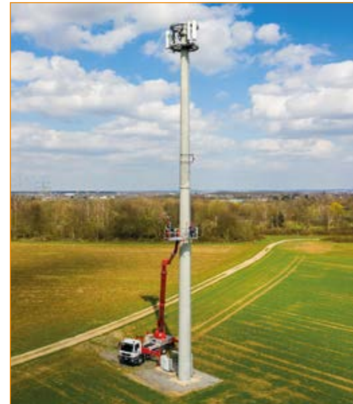
Left: The Ruthmann LES 100 Lifting Eye System allows e.g. also the assembly of the components behind projecting edges by means of the four possible assembly points.
